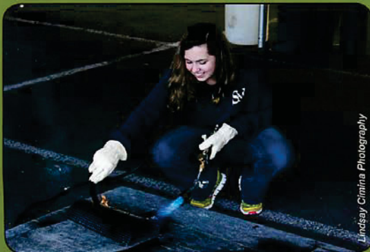
A career seeker learns the 'torch down' technique in a workshop with the NW Roofers & Waterproofers JATC
