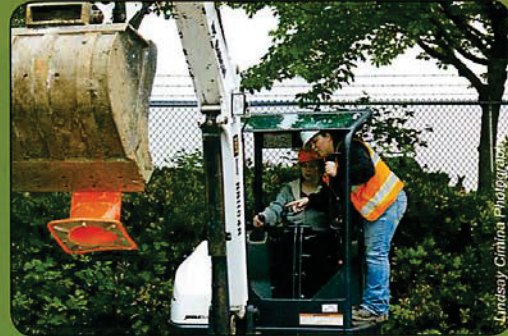
A high school student learns to operate heavy equipment in a workshop with Goodfellow Bros.
