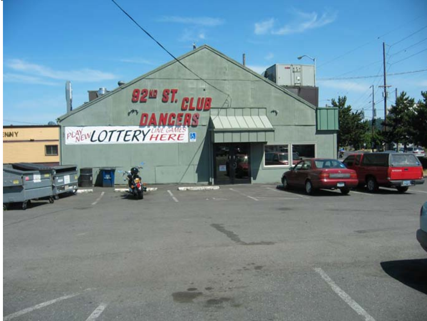
Property acquisition of MT. SCOTT PK, Lots 3 and 4, Block 1.
