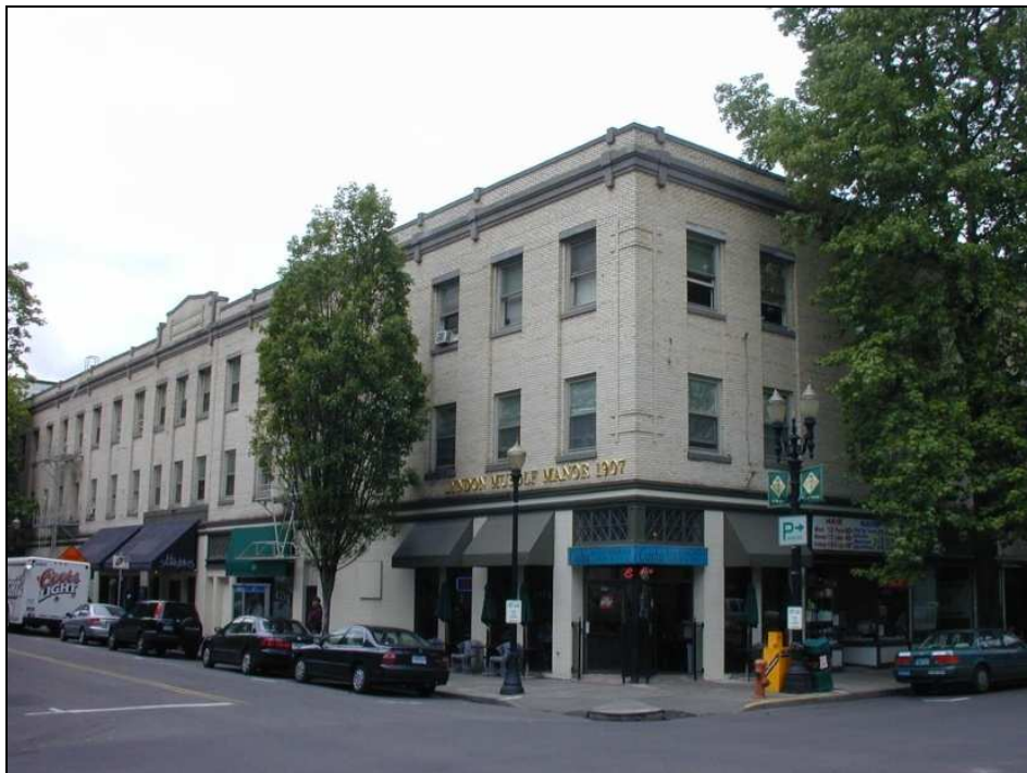
Musolf Manor's renovated housing for low income residents also has several improved commercial business spaces and has helped revitalize this corner in Old Town/China Town.
