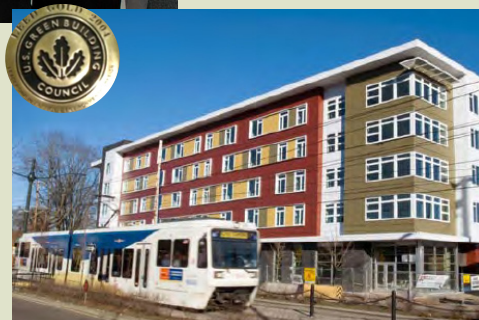
Located on the Interstate MAX light rail
