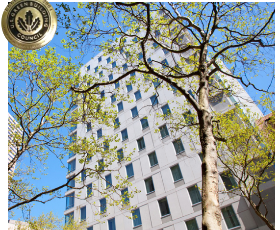
Portland City Center Courtyard Marriott received $600,000 in green build incentives for a total return on green investments of only 12 months.
