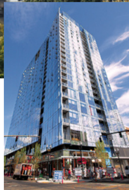
The Indigo @ twelve I west, a new mixed-use, luxury high-rise apartment building at SW 12th and Washington, is awaiting LEED Platinum certification. The new building is distinguished by four wind turbines mounted on the roof.
