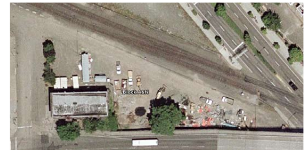
Aerial photo of Block A&N (prior to light rail construction)
