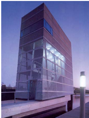
Wire Mesh Cladding Bridge Control Office, Netherlands
