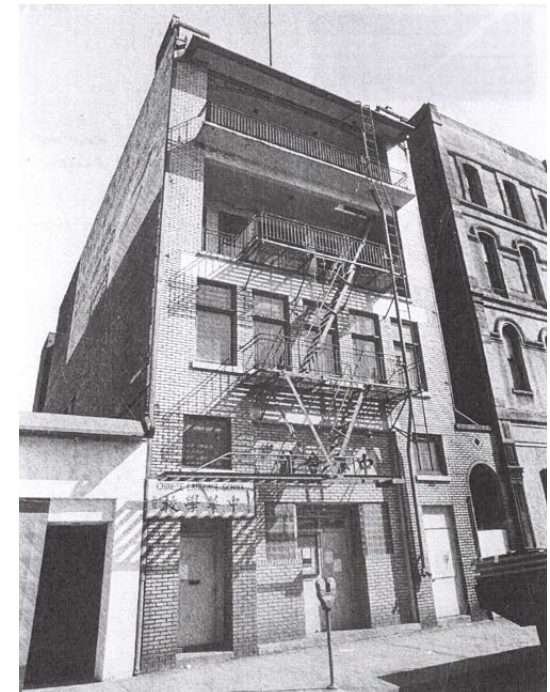
Archive photo of CCBA building, just south of the study area
