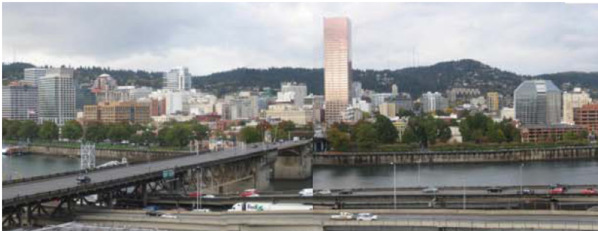
panoramic view of downtown portland from the burnside bridgehead site
