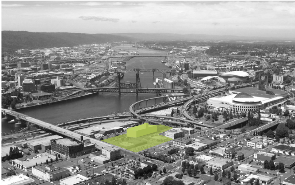
birdseye view of the burnside bridgehead looking west
